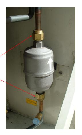
③Conduct vacuum-dehydrating from the quick joint located at the inlet side of dryer.
