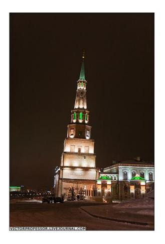
Suyumbike tower also refers to the "falling" towers (such as the Leaning Tower of Pisa), since it has a significant slope in the north-east. At the moment, its spire deviation from the vertical is 1.98 m.
