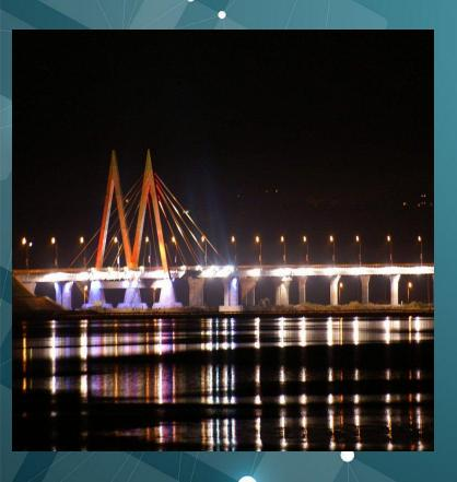
The modern bridge over the Kazanka river is more than one and a half kilometers long. The maximum height of the structure above water is 64 meters. Each side has three lanes and one footpath. The bridge was built by the Millennium of Kazan in 2005.
