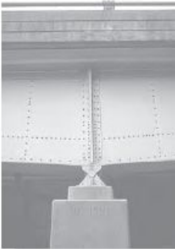
Pin support - Steel girder Railway bridge
