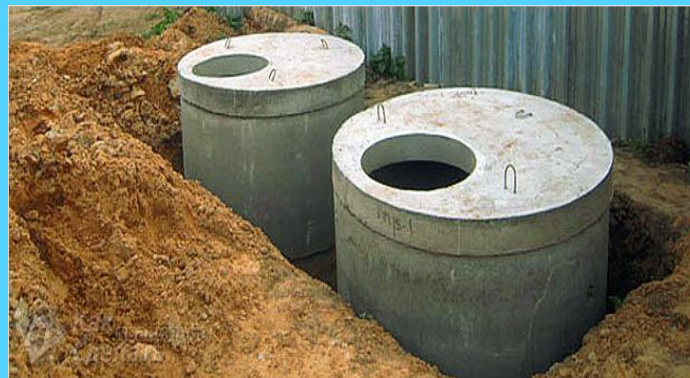
6. Tanks for TUZ drainage.
