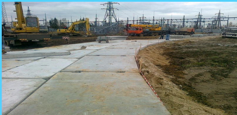
7. Concrete plates for infield roads.
