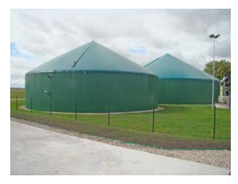
Biogas plant Vircava, Latvia 30 ton/day of maize silage Reactors 2400 m3 +1400 m3 CHP Deutz 600 KW el.
