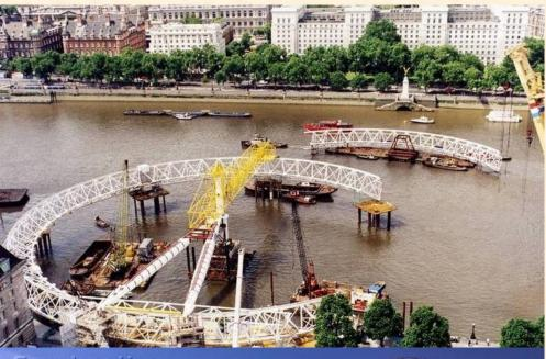
In the process over 1700 tons of steel were used for the structure and more than 3000 tons of concrete were used for the foundations. Its steel design forms an "A" shape, with two large tapered legs at the base -20 meters apart and each over 58 meters in length. The legs lean toward the river at a 65-degree angle. The rim of the Eye is supported by tensioned steel cables and resembles a huge spoked bicycle wheel.
