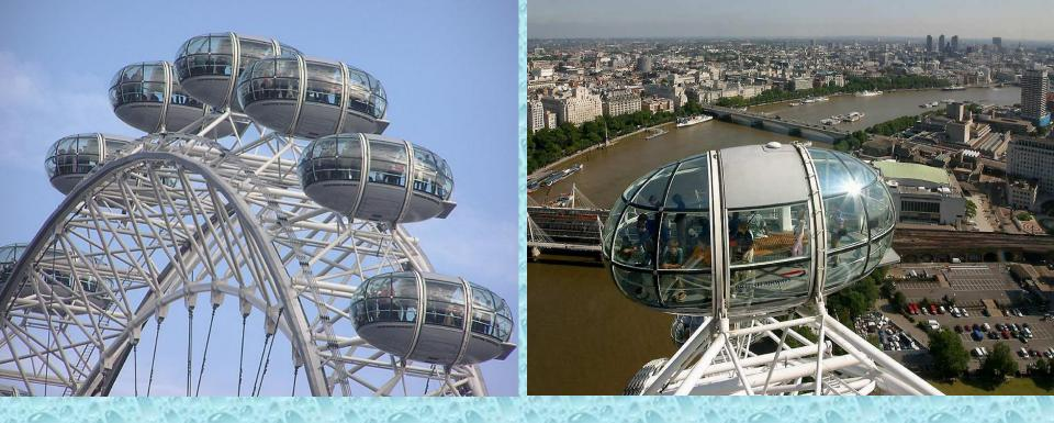
The wheel's 32 sealed and air-conditioned ovoidal passenger capsules are attached to the external circumference of the wheel and rotated by electric motors. Each of the 10-tonne capsules represents one of the London Boroughs, and holds up to 25 people, who are free to walk around inside the capsule, though seating is provided. The wheel rotates at 26 cm per second so that one revolution takes about 30 minutes.
